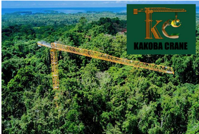
Binatang Research Centre Kakoba Crane commissioned in 2018
