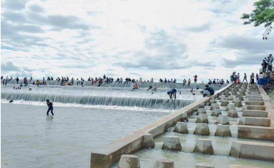
Figure 9: Cone design fish-way, Souy Weir (photo taken shortly after public opening) (A. O'Brien)
