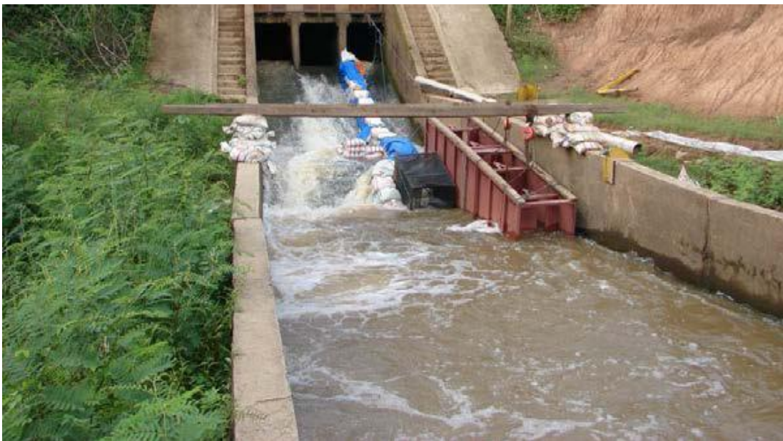
Figure11: Pak Peung Regulator with submerged temporary experimental orifice fishway for fish counting (Singhanouvong et al., 2015)
