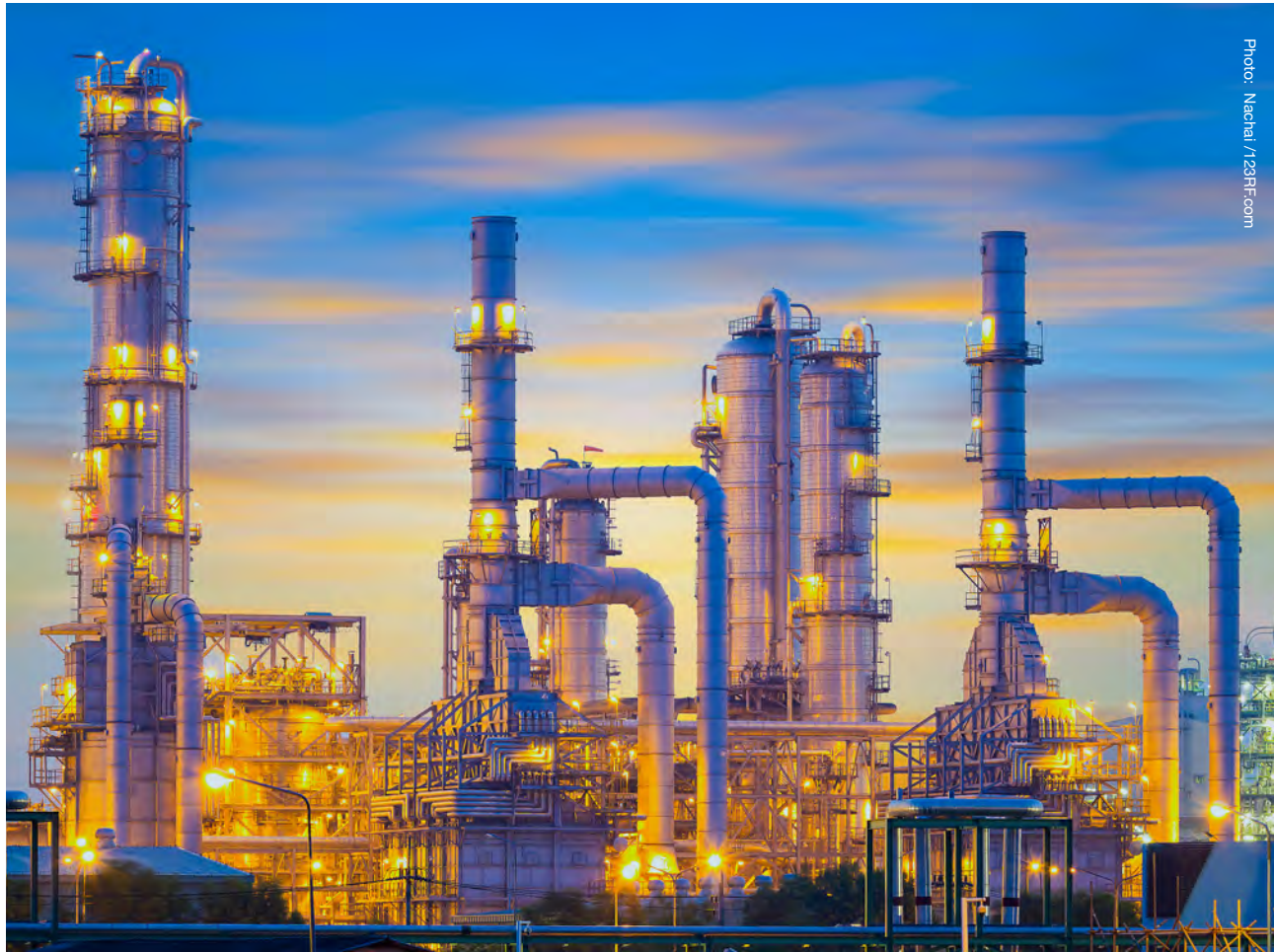
Companies in the oil and gas sector account for around 70% of all NDT inspection business in Malaysia (Photo: Nachai/123RF.com).
