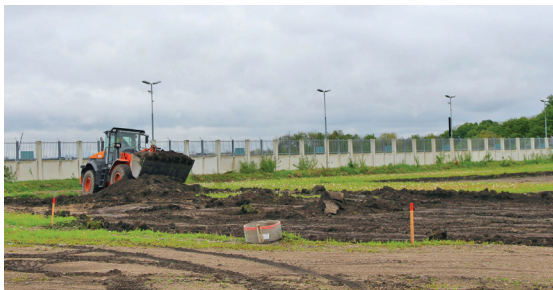
The start of excavation works for the FML
