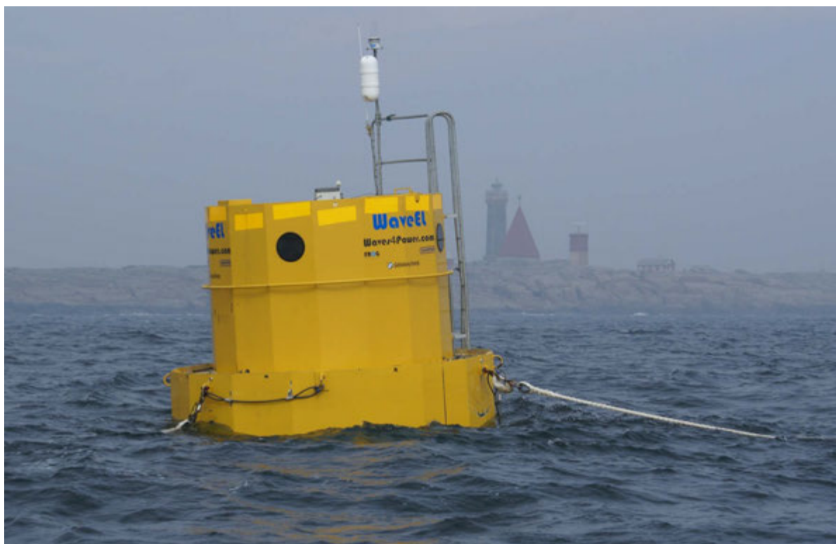
Figure 2. Waves4power OWC plant in operation offshore Sweden (Reprinted with permission from Waves4power AB).
