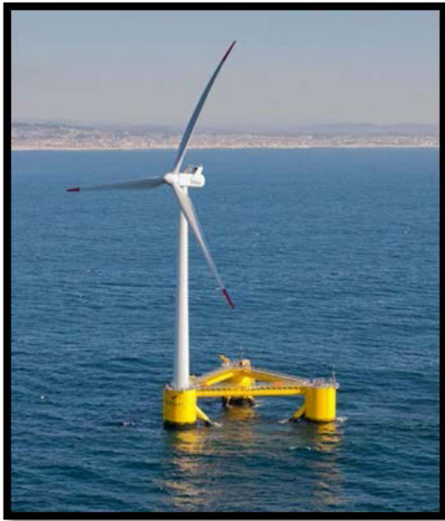
Figure 1. Photo credit: Principle Power. The WindFloat Prototype (WF1) floating wind turbine, deployed by Principle Power in 2011, 5km off the coast of Aguçadoura, Portugal. The WF1 is outfitted with a Vestas v80 2.0 MW offshore wind turbine. As of December 2015, the system has produced in excess of 16 GWh of renewable energy delivered to the local grid.
